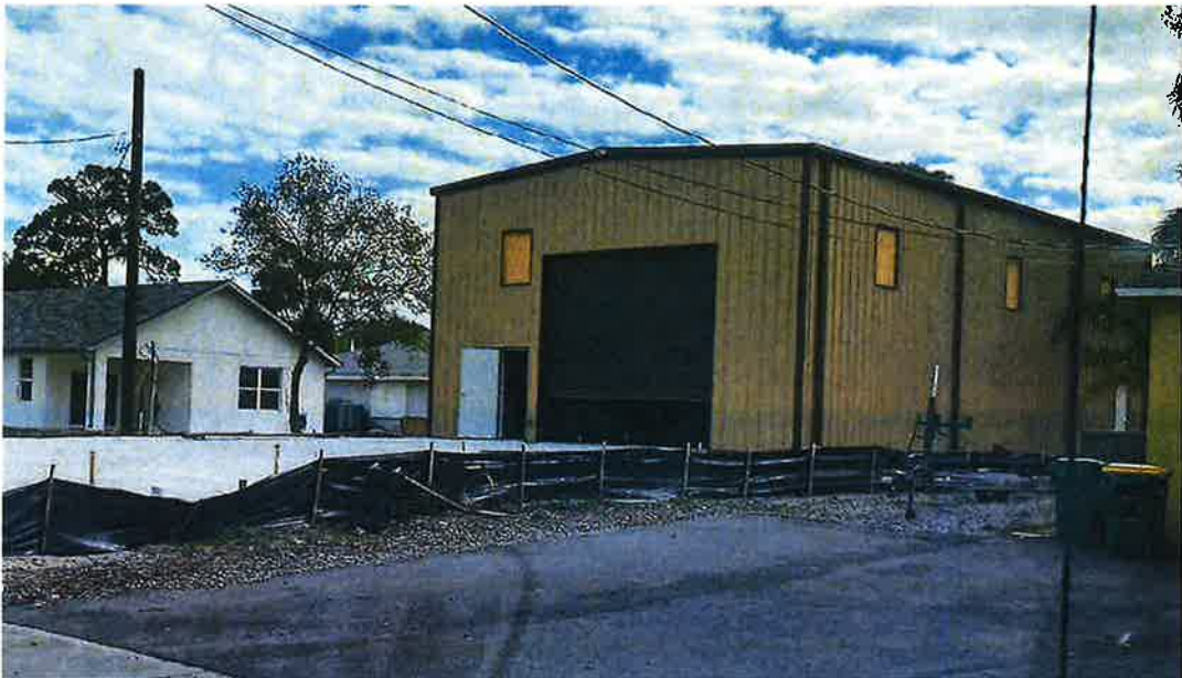
Note inclusion of high-bay door; absence of brick veneer
