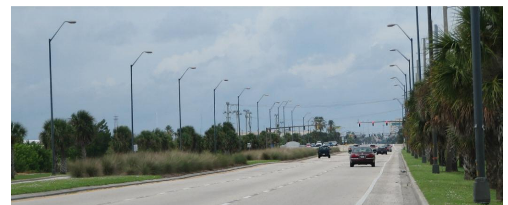
SR 520 East With Landscaping
