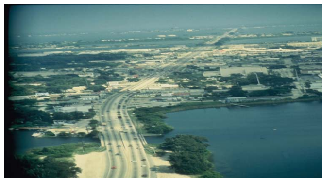
SR 520 prior to widening
