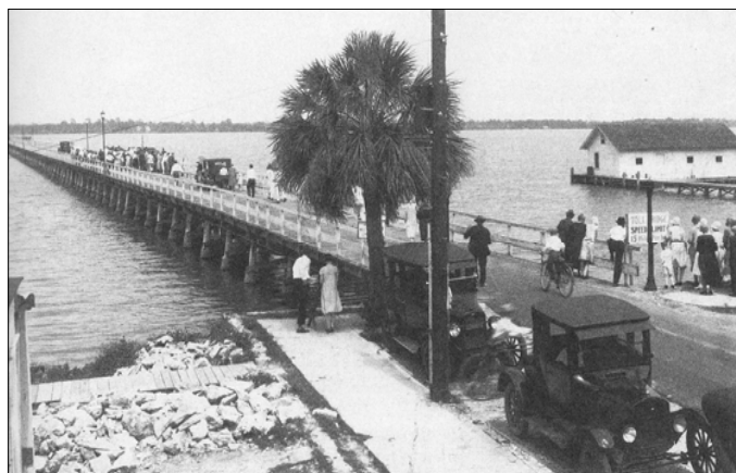
Opening of the first bridge between Cocoa and Merritt Island 1917
