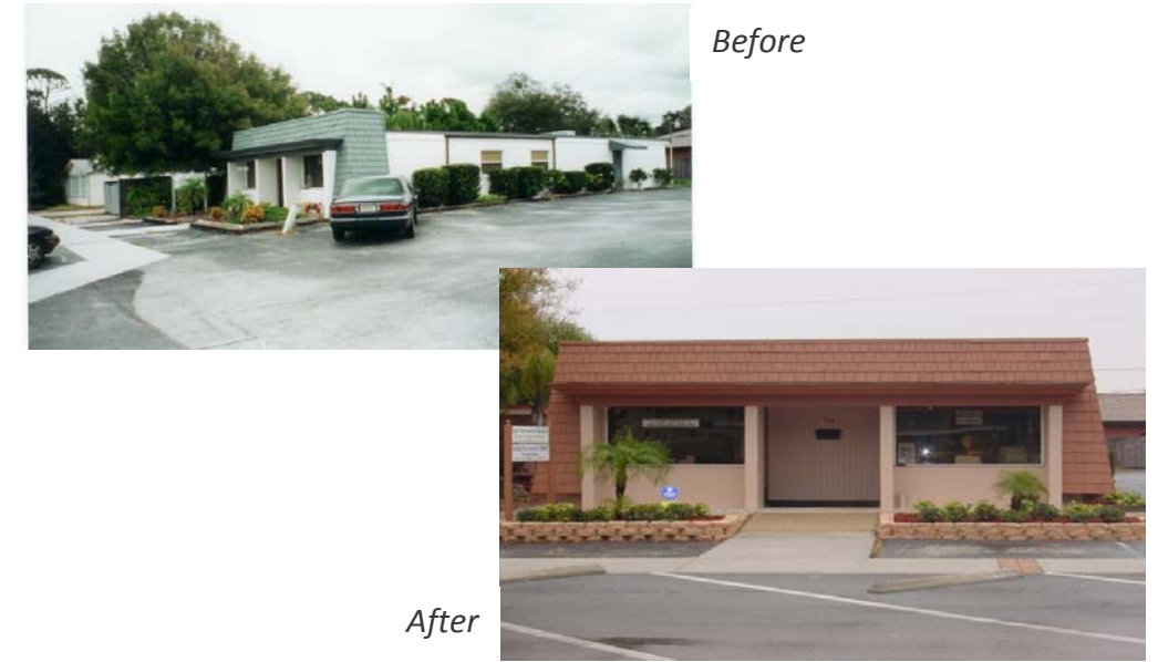
30 North Grove Street
